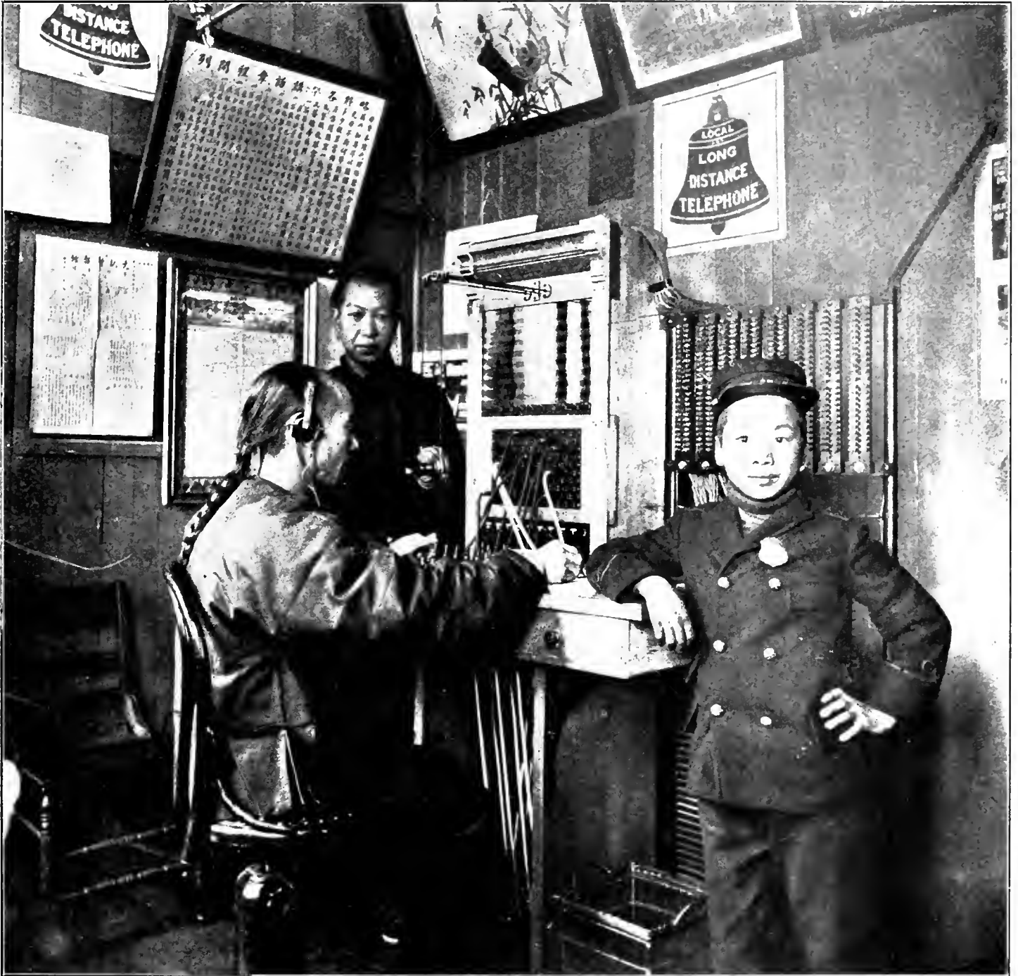
THE SAN FRANCISCO CHINESE TELEPHONE EXCHANGE IN 1897
